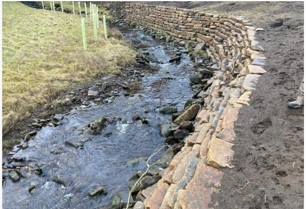
Example of interventions delivered through WAMM project to stabilise spoil heaps and prevent their erosion by the watercourse.
